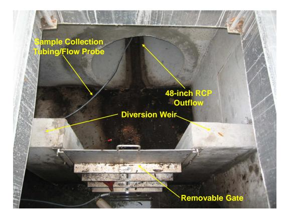
Figure 2-6. Interior of Diversion Structure.
