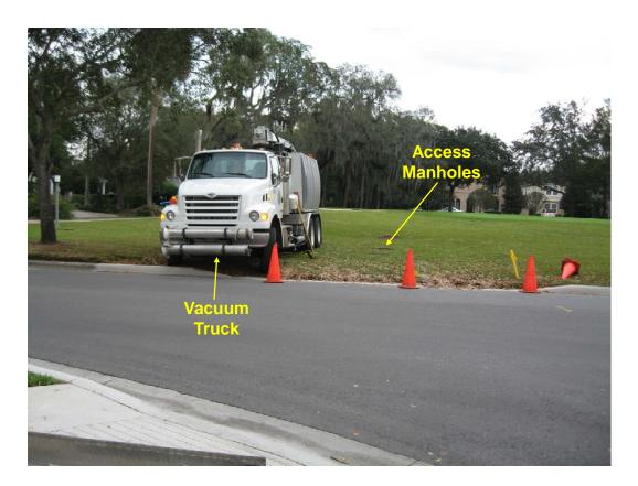
Figure 2-10. Cleaning Operations for the Screening Structure.
