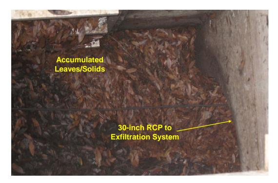
Figure 2-7. Accumulation of Leaves Inside the Diversion Structure.
